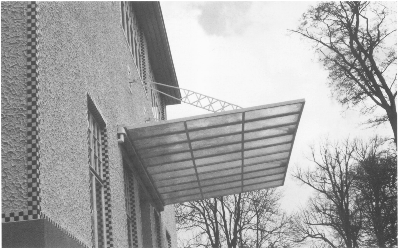
FIGURE 23: Josef Hoffmann, Purkersdorf Sanatorium, Purkersdorf, Austria, 1904–1905, restored 1995, close-up of canopy showing girder
